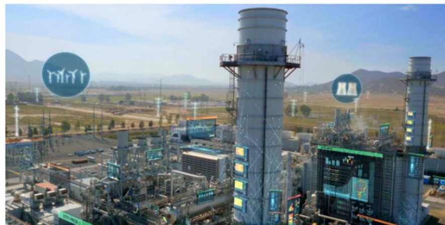
The digital power plant is one of Industrial Internet applications. Image credit: GE Power
